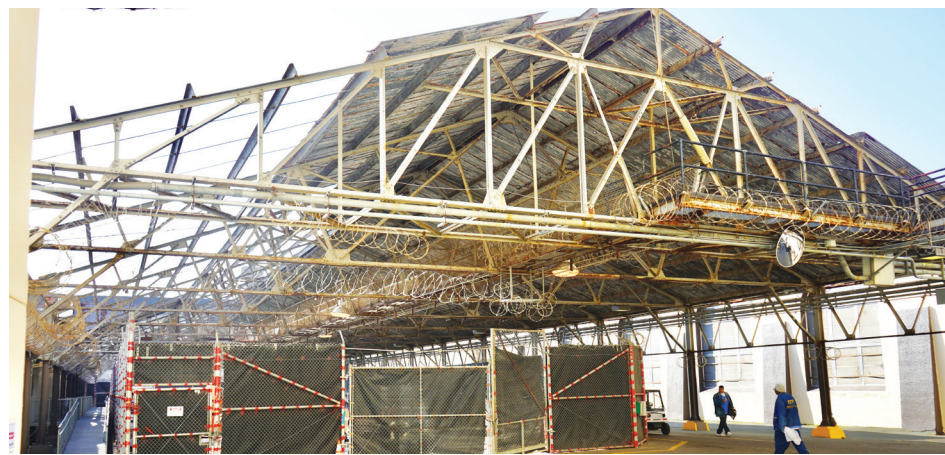
Upper Yard demolition removed isolation cells and amenities
